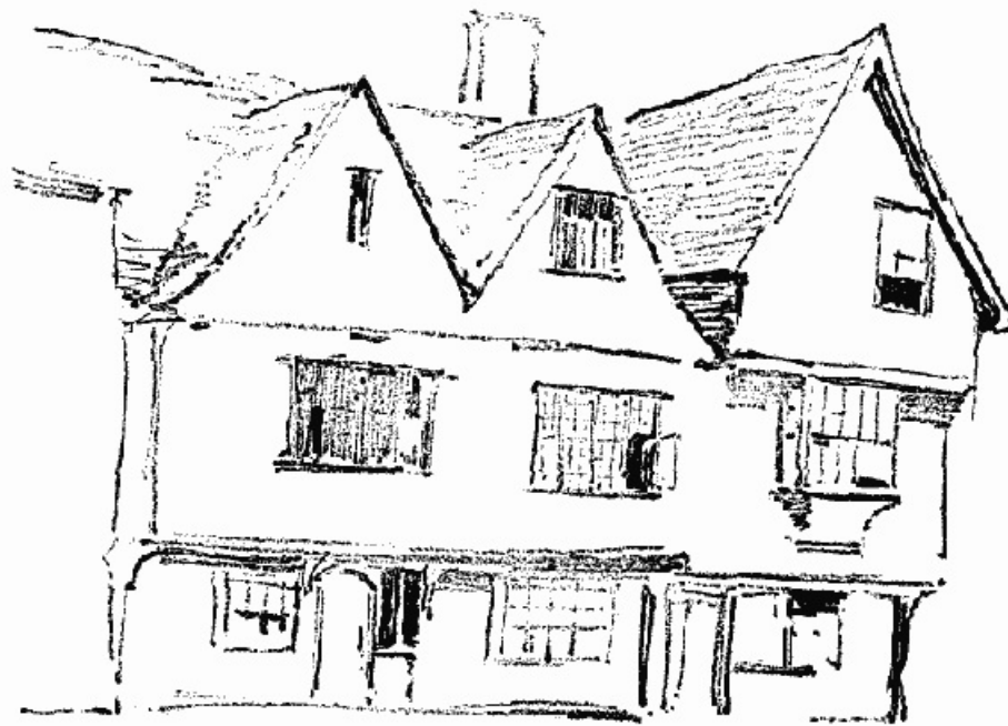
Tudor House, Ipswich, near the Custom House
