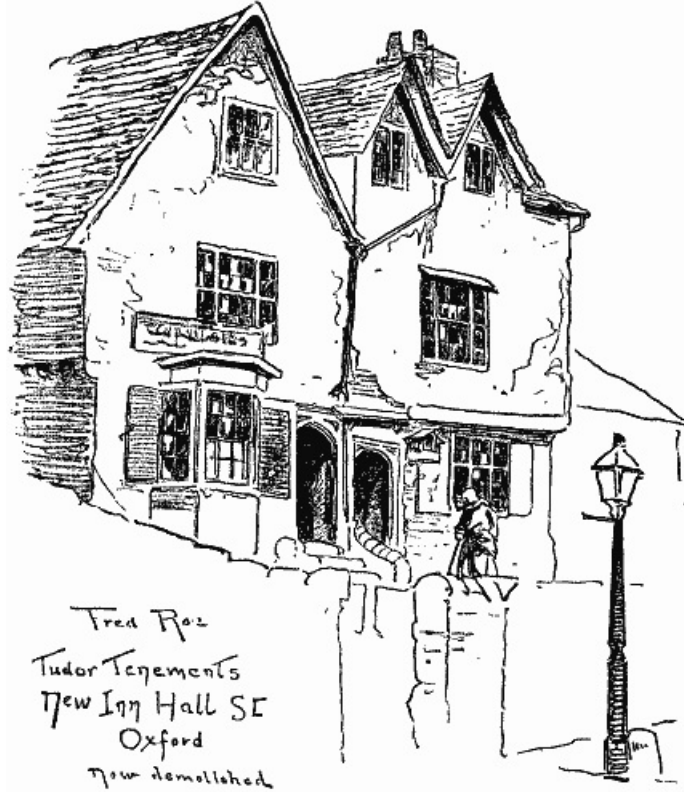
Tudor Tenements, New Inn Hall St, Oxford. Now demolished.
